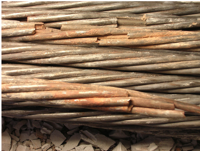
Figure 4-75: Corrosion under the load point - Specimen 9
