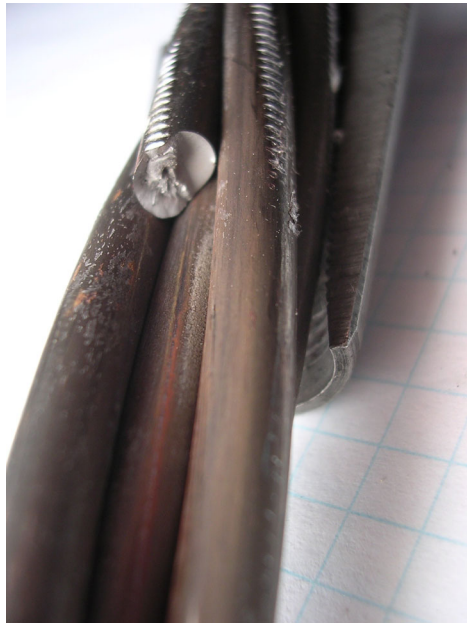
Figure 4-63: Wire break on strand 9 at deck end
