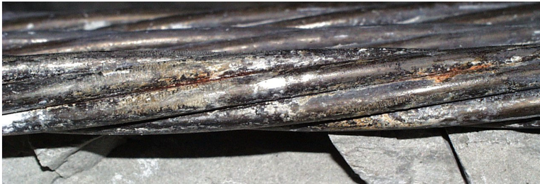
Figure 4-21: Corrosion on Strand 19 near tower anchor head - Specimen 6
