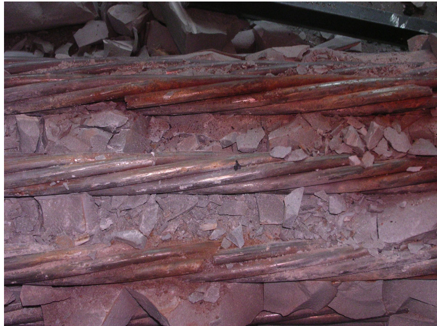
Figure 4-92: Corroded fretting product at the tower end - Specimen 10
