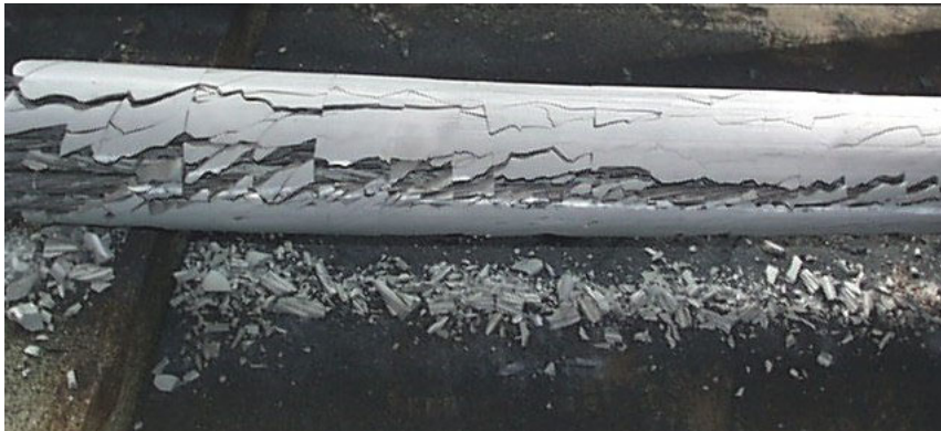
Figure 4-89: Grout at midspan immediately after opening - Specimen 10
