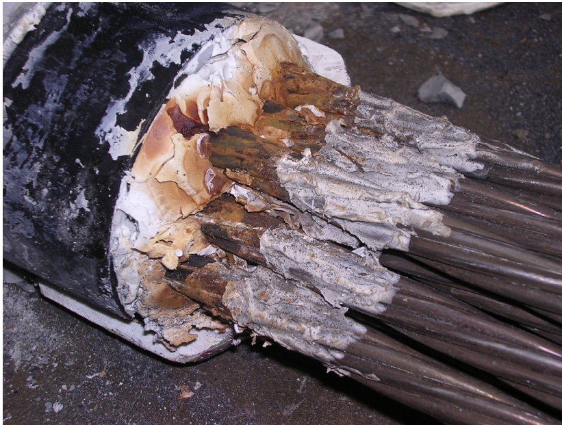
Figure 4-57: Corrosion at interface between strand and caulk - Specimen 8
