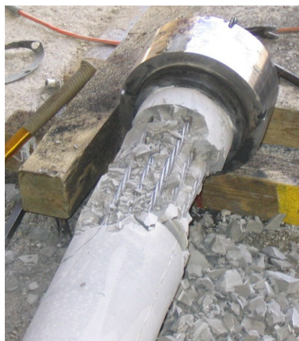
Figure 4-36: Condition of grout at deck anchor head several minutes after removing polyethylene pipe - Specimen 7
