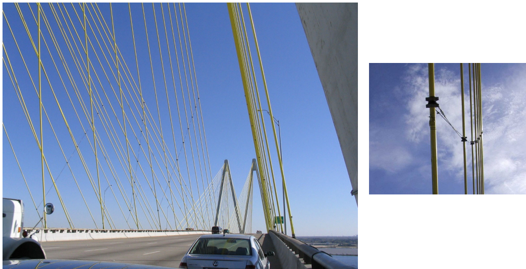
Figure 1-4: Cable restrainers on bridge
