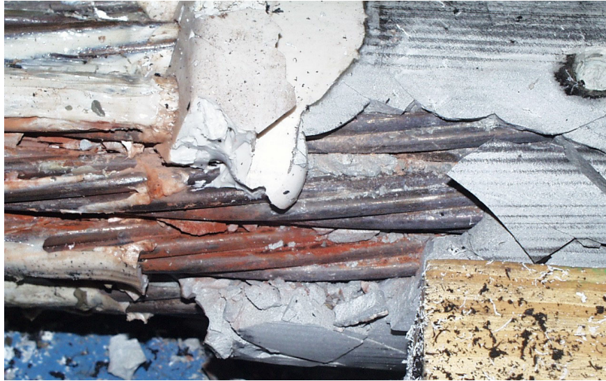
Figure 4-10: Interface between caulk and grout – Specimen 5
