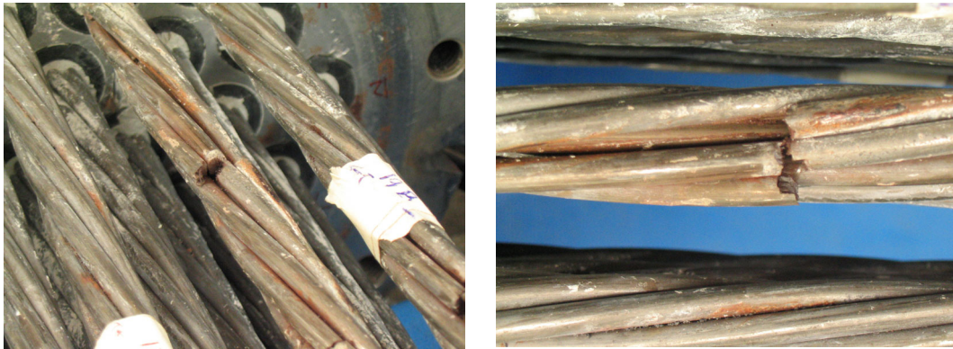
Figure 4-38: Corrosion found near anchorage on strand 18 - Specimen 7
