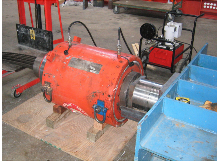
Figure 2-15: Setup for stressing
