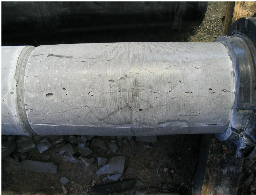
Figure 4-34: Grout condition at tower end - Specimen 7
