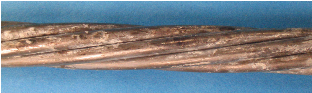
Figure 4-40: Corrosion on strand 17 at midspan - Specimen 7
