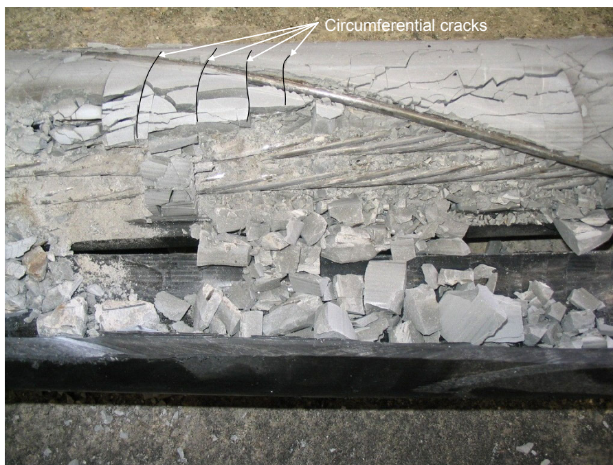
Figure 4-37: Grout condition under load point - Specimen 7
