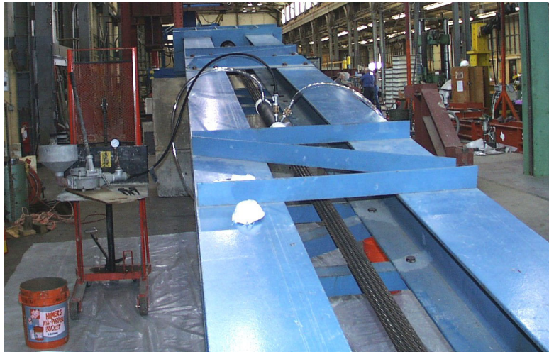
Figure 2-18: Grouting setup for Specimen 8
