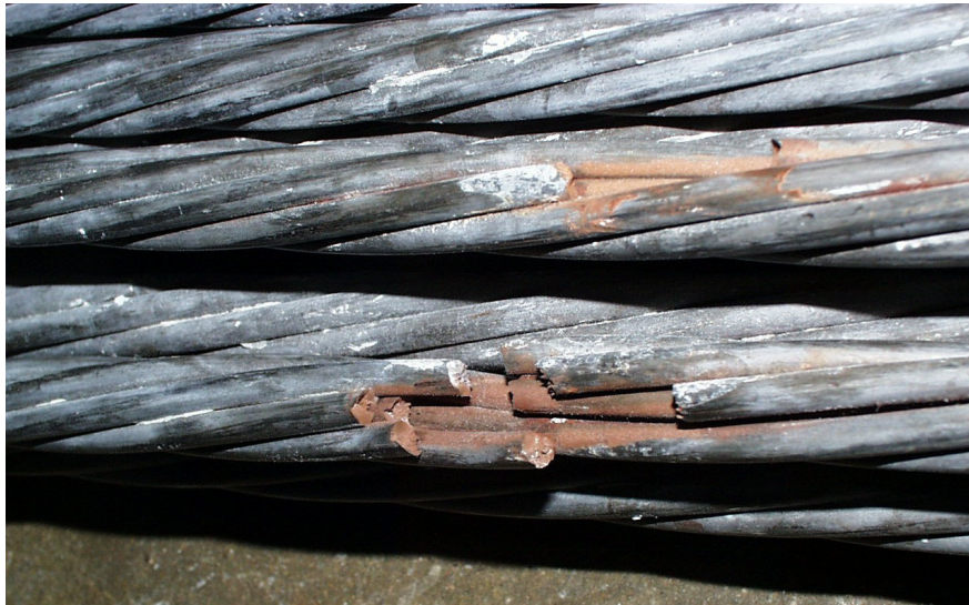
Figure 4-91: Corroded fretting product under the load point – Specimen 10
