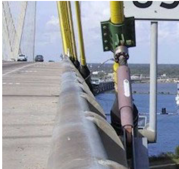
Figure 1-5: Dampers installed by WDP
