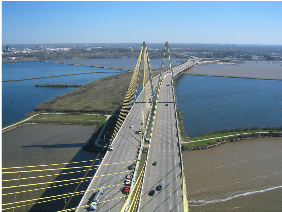
Figure 1-2: Two independent decks of the Fred Hartman Bridge
