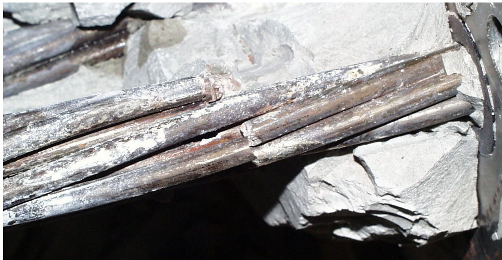
Figure 4-26: Wire breaks on strand 1 near the tower anchor head - Specimen 6
