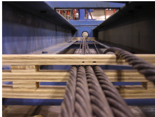
Figure 2-9: Wood shelf used to separate strands during construction
