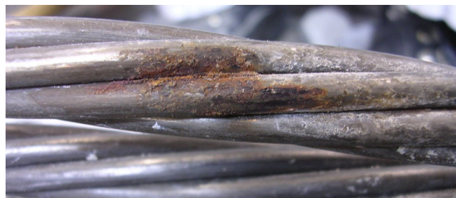
Figure 4-74: Corrosion near the tower anchorage - Specimen 9
