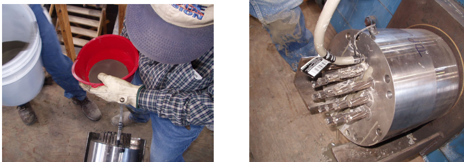
Figure 2-25: Filling of grout void near tower anchor head
