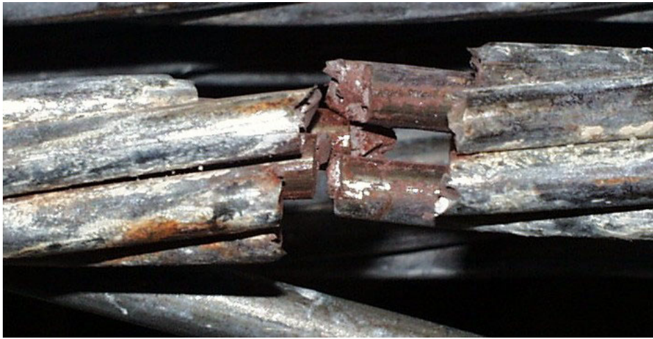
Figure 4-20: Corroded fretting product on Strand 19 – Specimen 6
