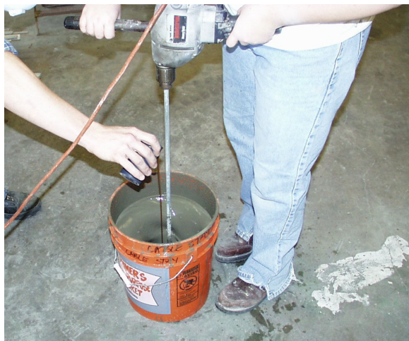
Figure 2-19: Grout mixing using electric drill and paddle mixer
