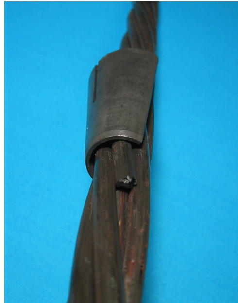
Figure 4-64: Wire break on strand 11 at deck end
