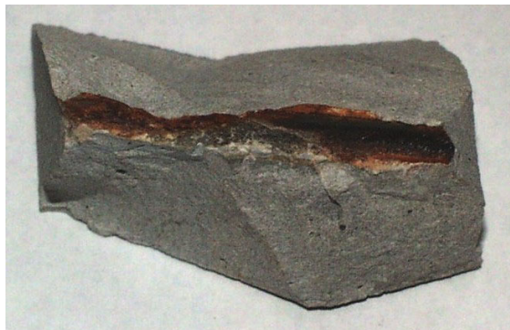
Figure 4-22: Corrosion product on grout from tower end - Specimen 6
