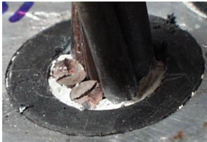
Figure 4-27: Wire breaks on strand 17 at the face of the tower anchor head - Specimen 6
