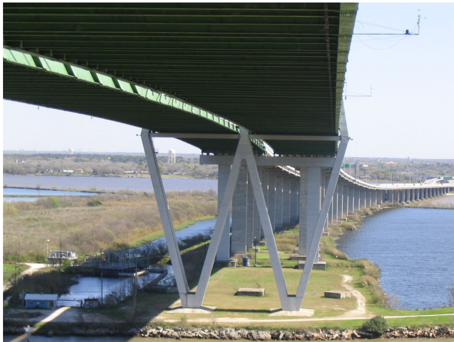
Figure 1-3: Point at which bridge towers are joined
